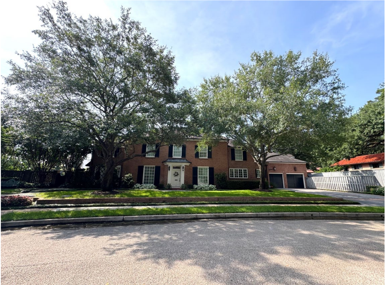
Photo 3: Zoomed out view of the north (front) elevation of the Dr. and Mrs. Robert A. Johnston House and garage. Camera facing south. Photo by HOP staff Cara Quigley, July 2024.
