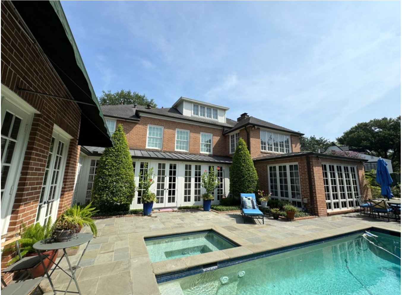
Photo 12: Oblique view of the south (rear) elevation of the Dr. and Mrs. Robert A. Johnston House. Camera facing northeast. Photo by HOP staff Cara Quigley, July 2024.
