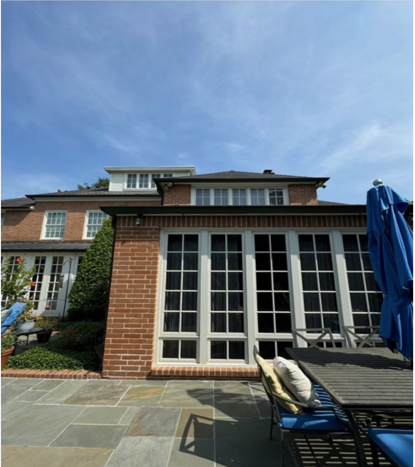
Photo 10: South (rear) elevation of the Dr. and Mrs. Robert A. Johnston House. Camera facing north. Photo by HOP staff Cara Quigley, July 2024.
