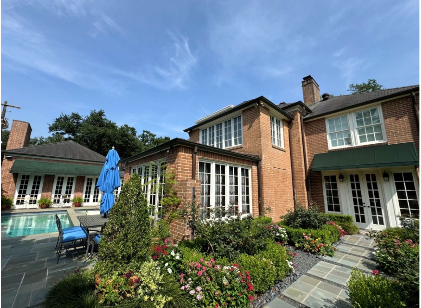
Photo 9: Oblique view of the south (rear) elevation of the Dr. and Mrs. Robert A. Johnston House. Camera facing northwest. Photo by HOP staff Cara Quigley, July 2024.
